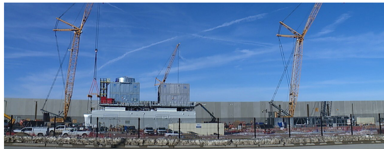
IN THE PHOTO CONSTRUCTION AT A GOOGLE DATA CENTER CAMPUS IN NORTHLAND KC, BRIAN LINTON/41 KSHB
